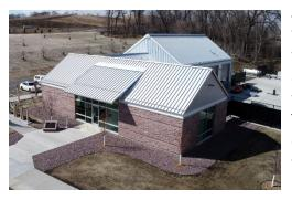
Administrative/Maintenance Facility: The building was constructed with a standard wood roof trusses with a detailed overhang to accommodate the architect's aesthetic vision. The walls were framed with wood studs and cladded with quartzite stone. The Maintenance building was constructed as Preengineered Metal Building (PEMB). Heyer worked with the manufacturer to coordinate the link between buildings and associated concrete foundations.
