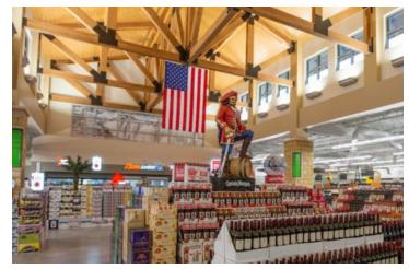
mezzanine area is comprised of standard wood scissor trusses. The remainder of the retail and storage area roof framing is standard metal deck and steel joist framing with a fully adhered membrane roof.
